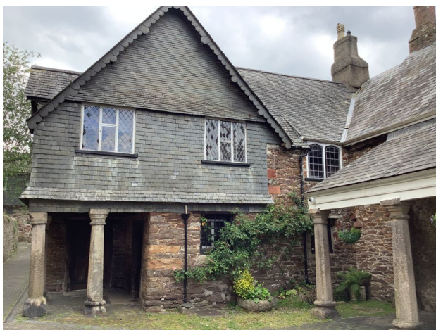
Guildhall Cottage, rear St. Mary's Church
